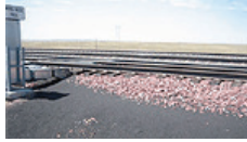
Note coal dust accumulation alongside track Enlarge
