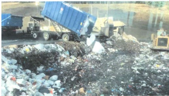
Tipping of typical industrial tote bags of wastes from Republic tip trailer. Note "white" layer on compacting dozer (right side of photo).
